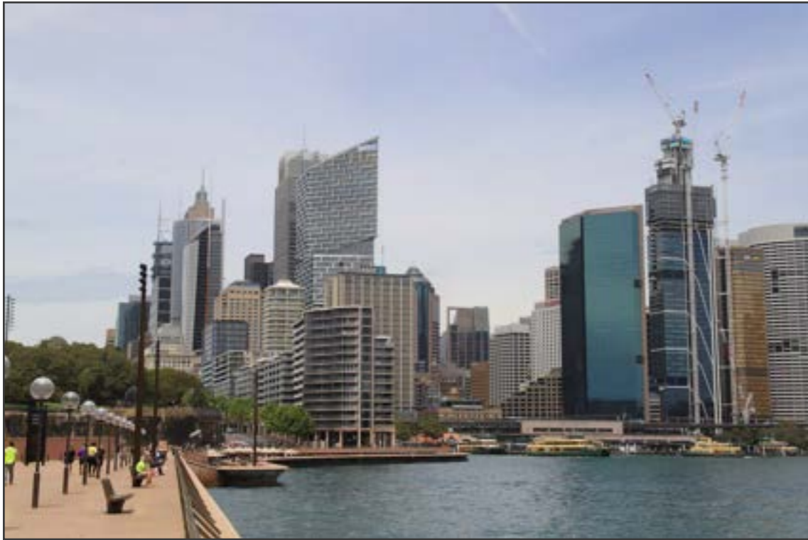
PHOTOGRAPH SHOWING CURRENT CONDITION
