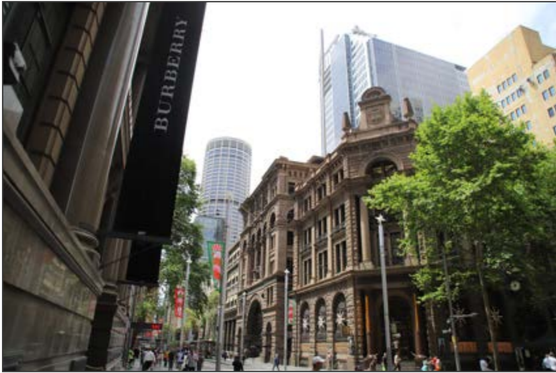
PHOTOGRAPH SHOWING CURRENT CONDITION
