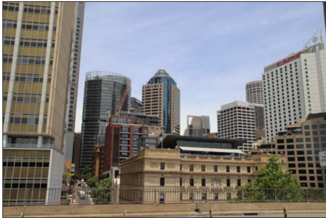
PHOTOGRAPH SHOWING CURRENT CONDITION
