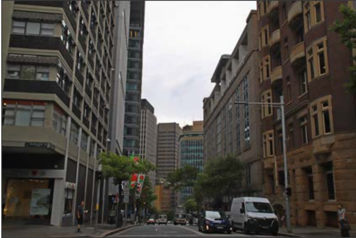
PHOTOGRAPH SHOWING CURRENT CONDITION
